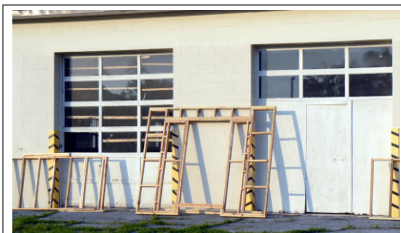
East Building: Frames ready to install!
