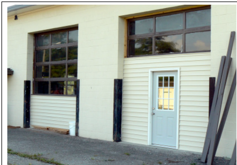
West Building: Old doors gone! New door installed!
