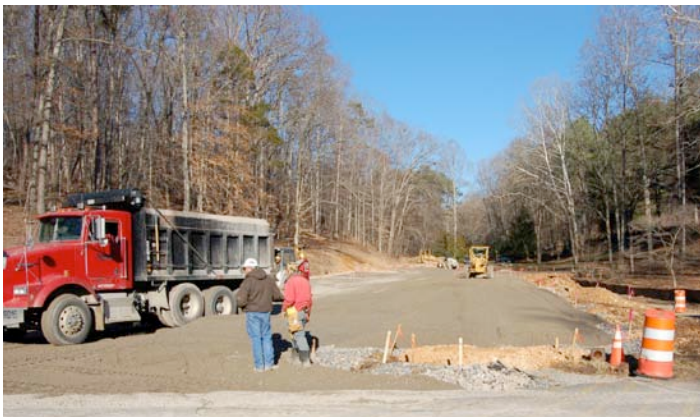
The new parking area nears completion
